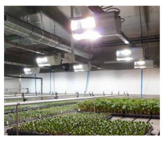
At Semillas Fitó, two germination chambers have been updated with a total of 18 new 250 W LED lamps, replacing the incandescent halide lamps which consumed 315 W each.
